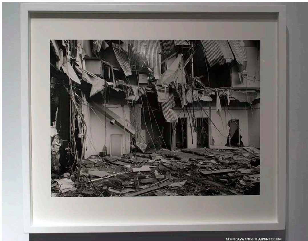
LaToya Ruby Frazier's UPMC Professional Building Doctor's Offices , 2011, from the series, "The Grey Area," which documents the demolition of Braddock Hospital in her Pennsylvania home town, which she had been involved in trying to save, as seen in All Power . Ms. Frazier's work in All Power were lent to the exhibition by Gavin Brown's Enterprise.
