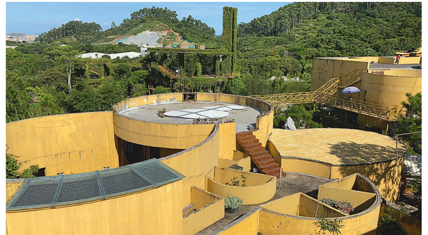
Rooftop view of the main architectural complex. The Museum of the Wind can be seen in the distance.
